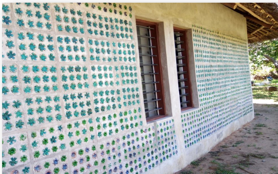
Plate 4.3: Wall built with plastic bottles.
