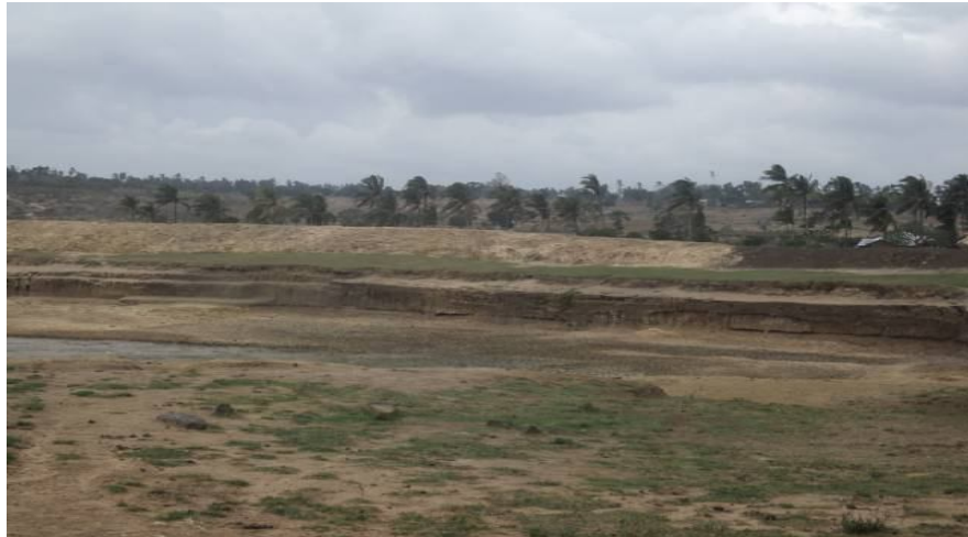
Figure 4.19: Dilapidated water pan in Kaya Fungo location
