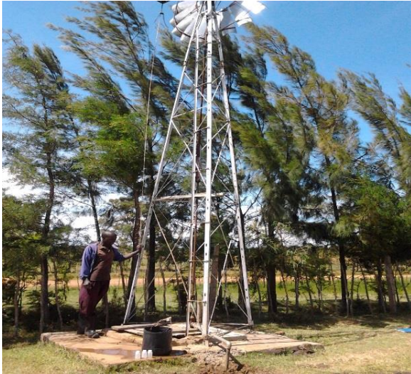
Plate 3: Protected wells within the medium farm sizes showing modes of water extraction of a windmill (left) and bucket/rope extraction methods (right).
