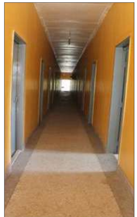
A corridor in one of the renovated Ruwenzori blocks
