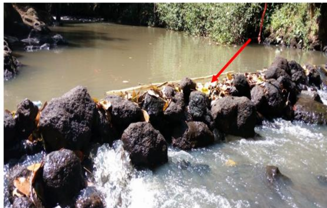
Plate 4: A photograph taken at Canning showing channel modification to create pools for watering livestock
