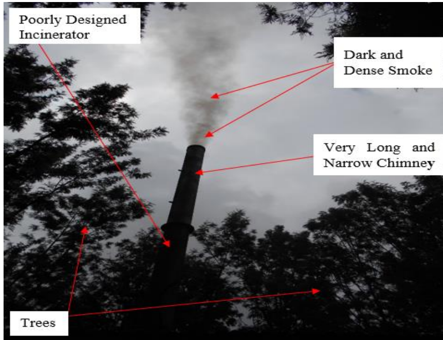
Plate 4.3: Dark and dense smoke at Community Resource Centre incinerator
