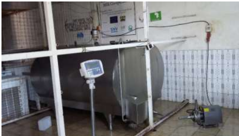
Appendix M: A horizontal milk cooler at a collection centre in Isiolo
