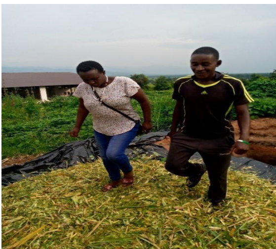
Figure 6: Filling and compacting the silo
