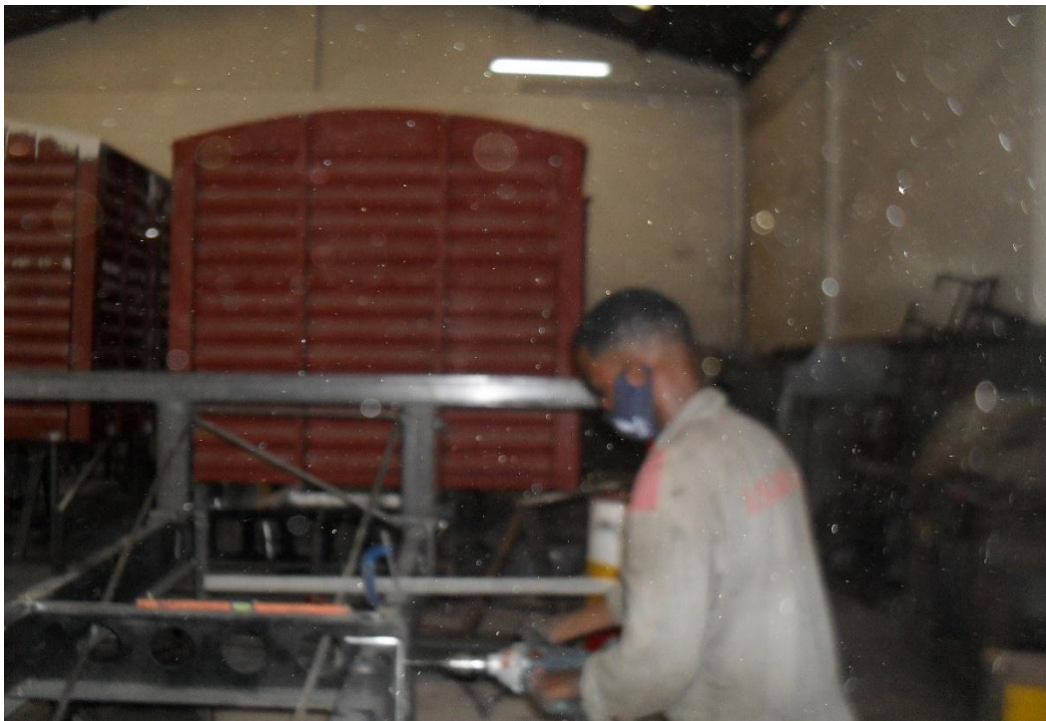
Plate 7: below shows a technician drilling points for mounting vehicle body in industry
