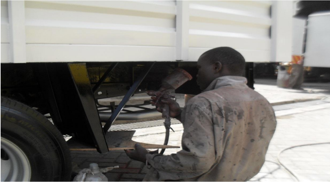
Plate 1, 2, and 3 vehicles spray painting in the manufacturing industry.
