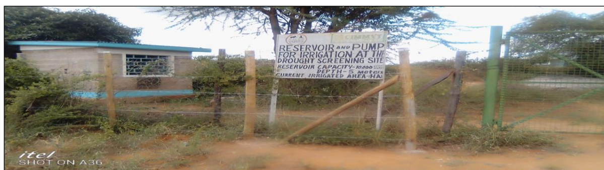
Plate 3. KALRO and CIMMYT water harvesting reservoir in Makueni County.
