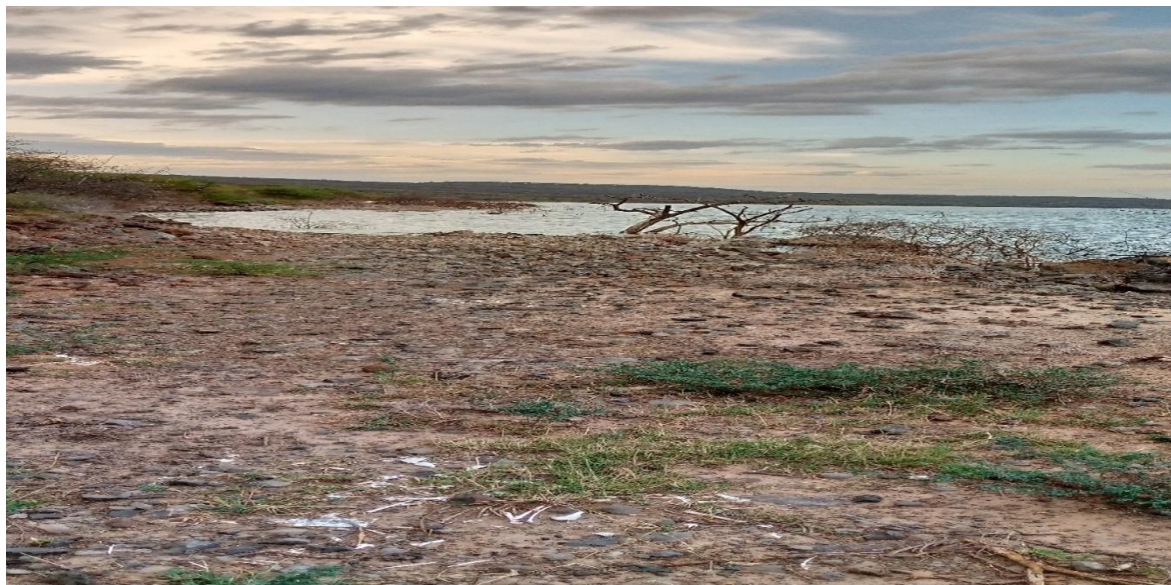
Plate 4.21: A Section of the Road Submerged Under Flood Water from Lake Bogoria
