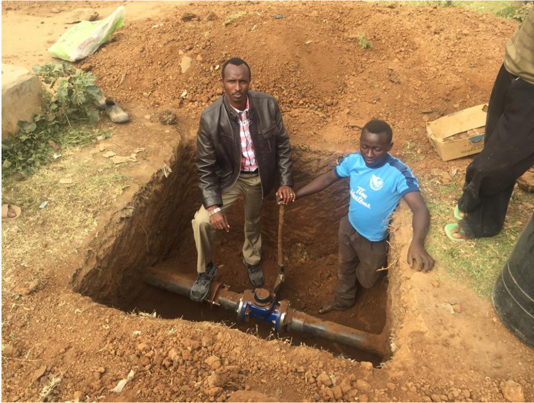
Figure 3.3: Installation of a Water Meter for Flow Measurement
