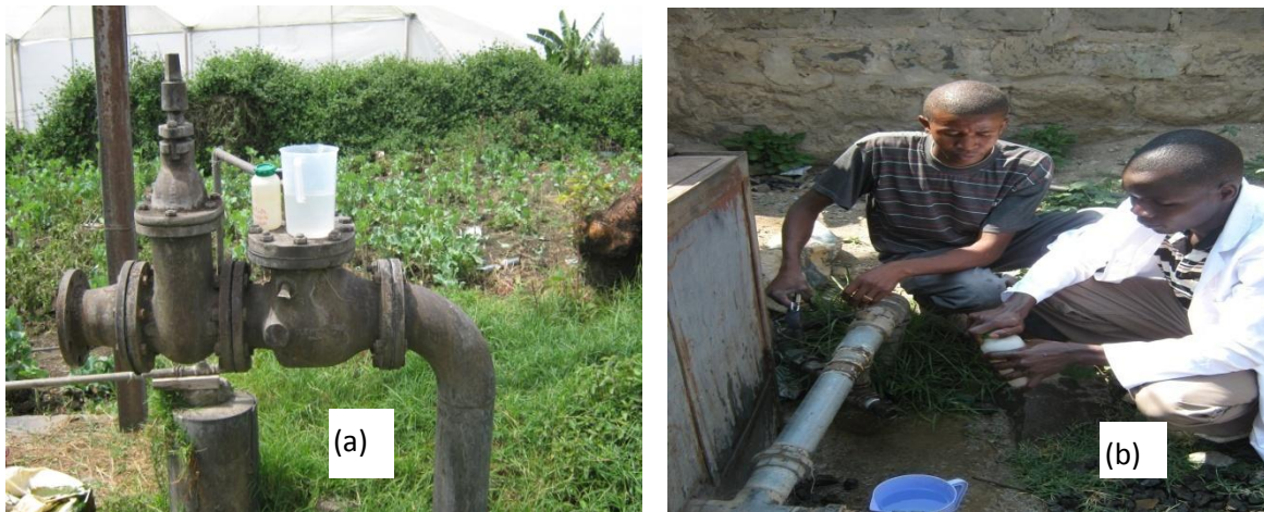
Plate 2: Direct borehole sites; (a) DCK and (b) KRBH III
