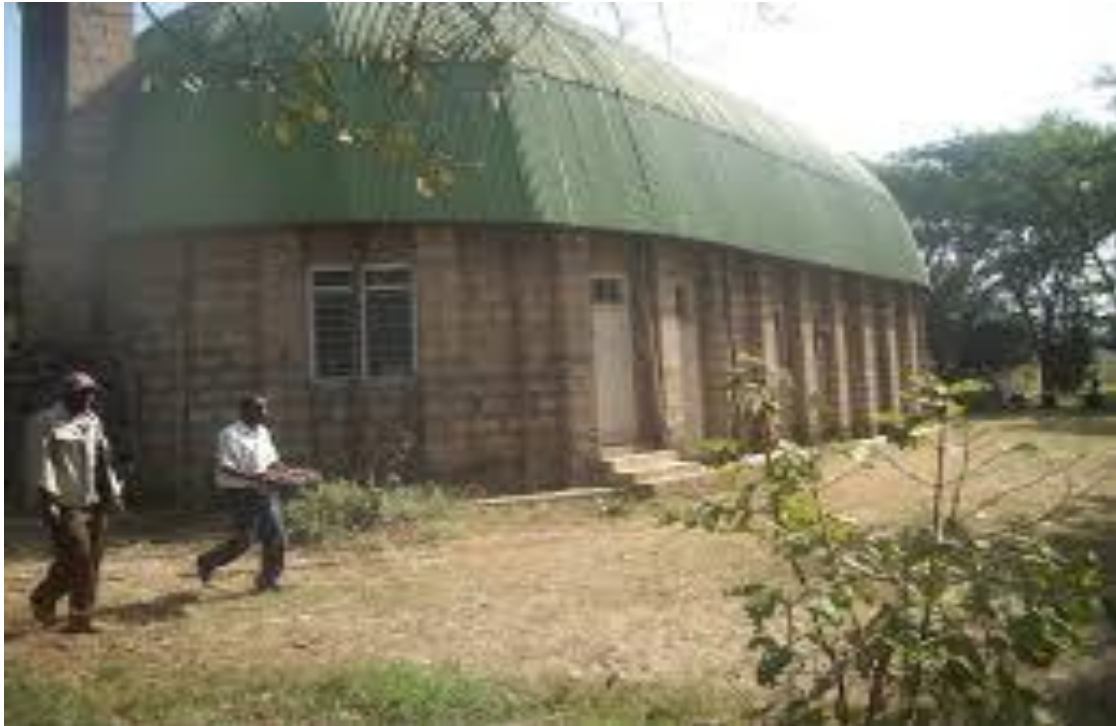
Plate 6: Njuri Ncheke shrine and the dome-shaped sacred hut.
