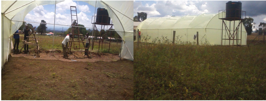
m) The greenhouse under construction
