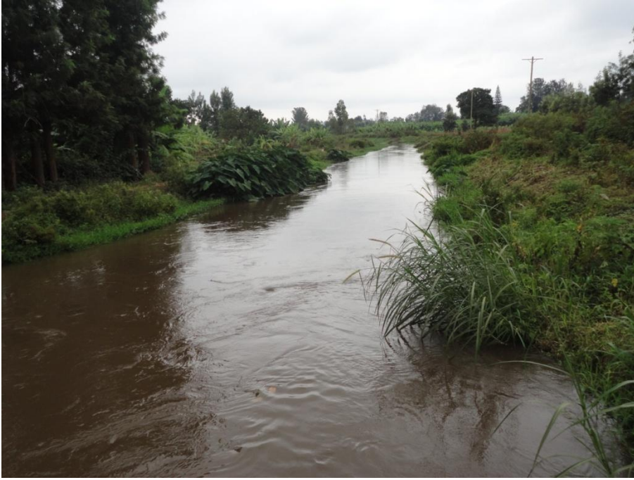
Figure 3.3: A section of Link canal II
