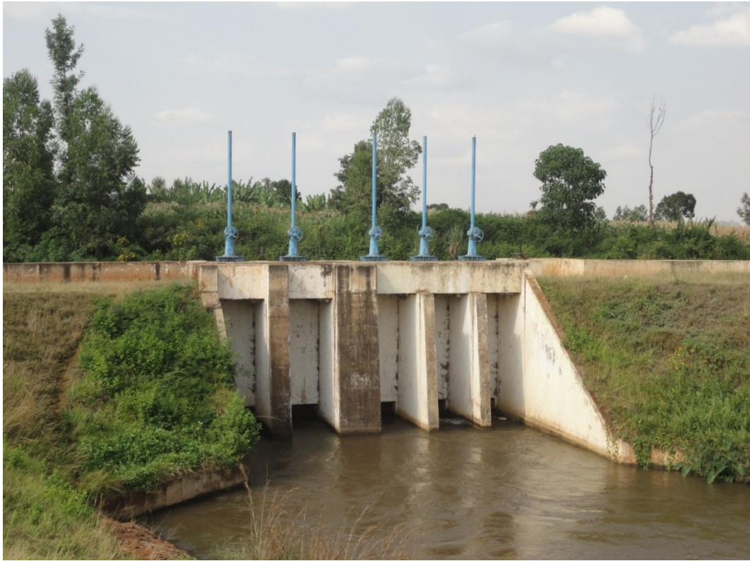
Figure 3.2: Upstream view of gates at Thiba off-take in MIS
