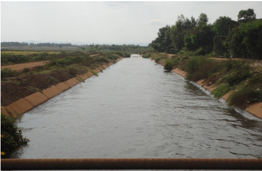
Figure 3.4: A section of lined trapezoidal Thiba Main Canal
