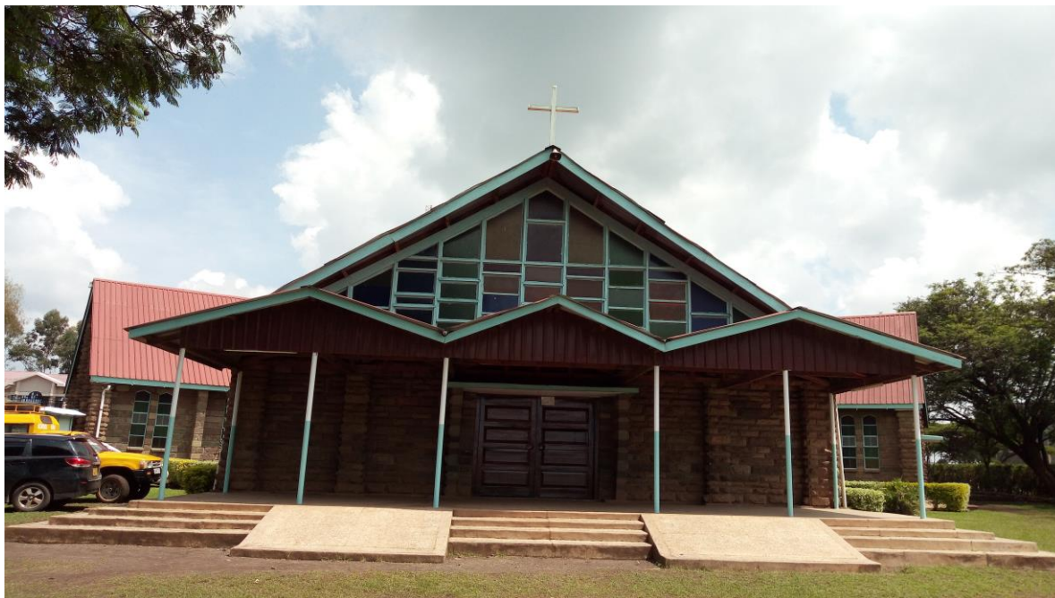
St. Lwanga Church building-Njoro
