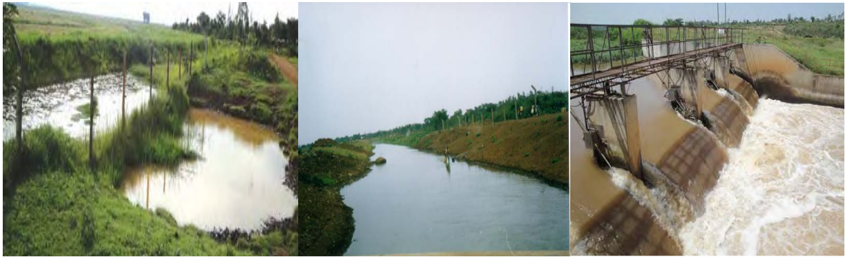
Water control methods: A Dyke (left); A Canal (centre); A Weir (right)
