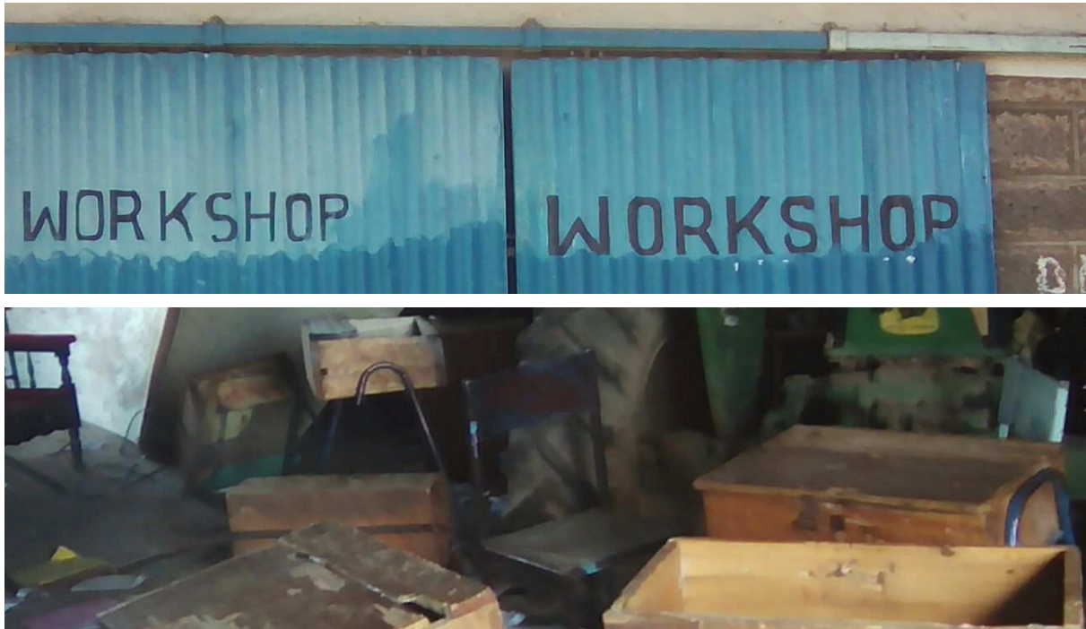
Figure 5: The status of the workshop in Narok high school
