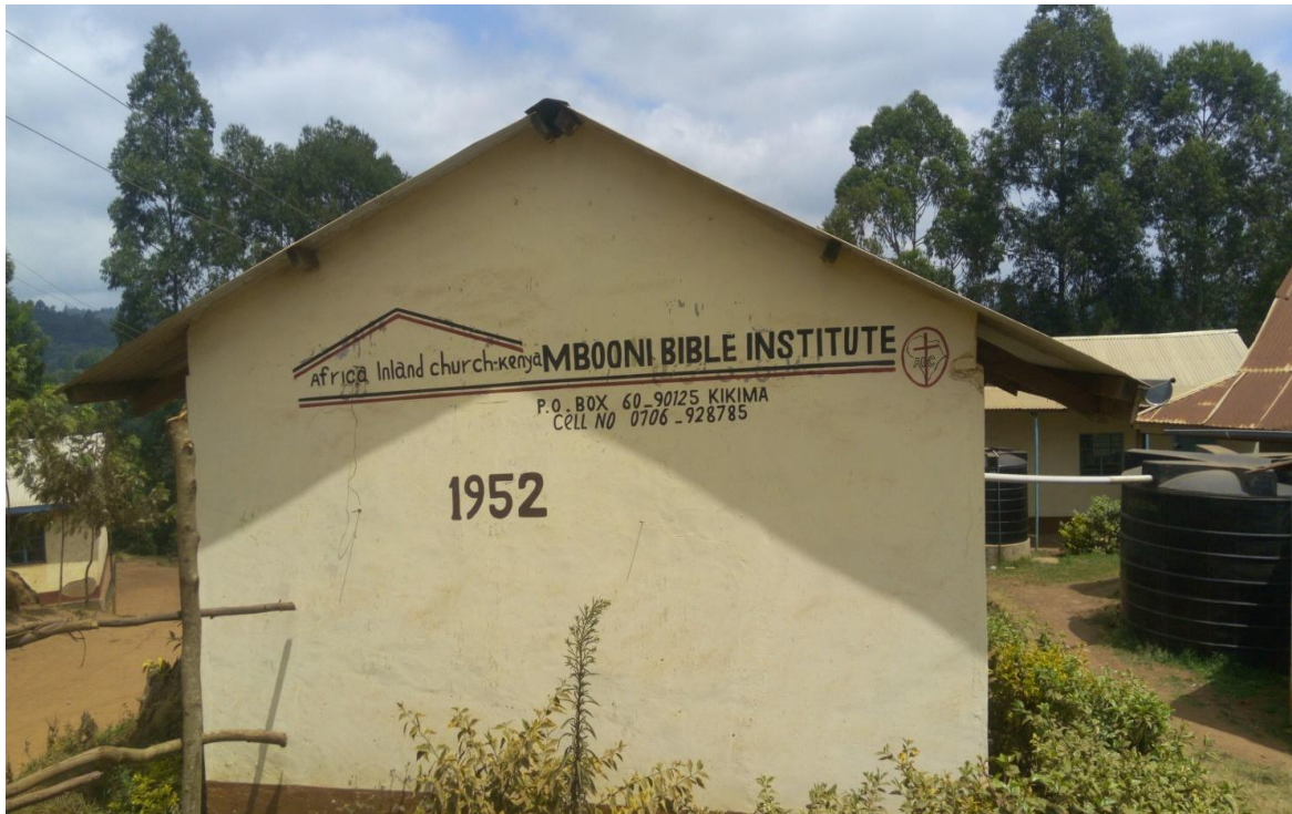
Figure 3.8 Some of the Structures of the Mbooni Bible Institute
