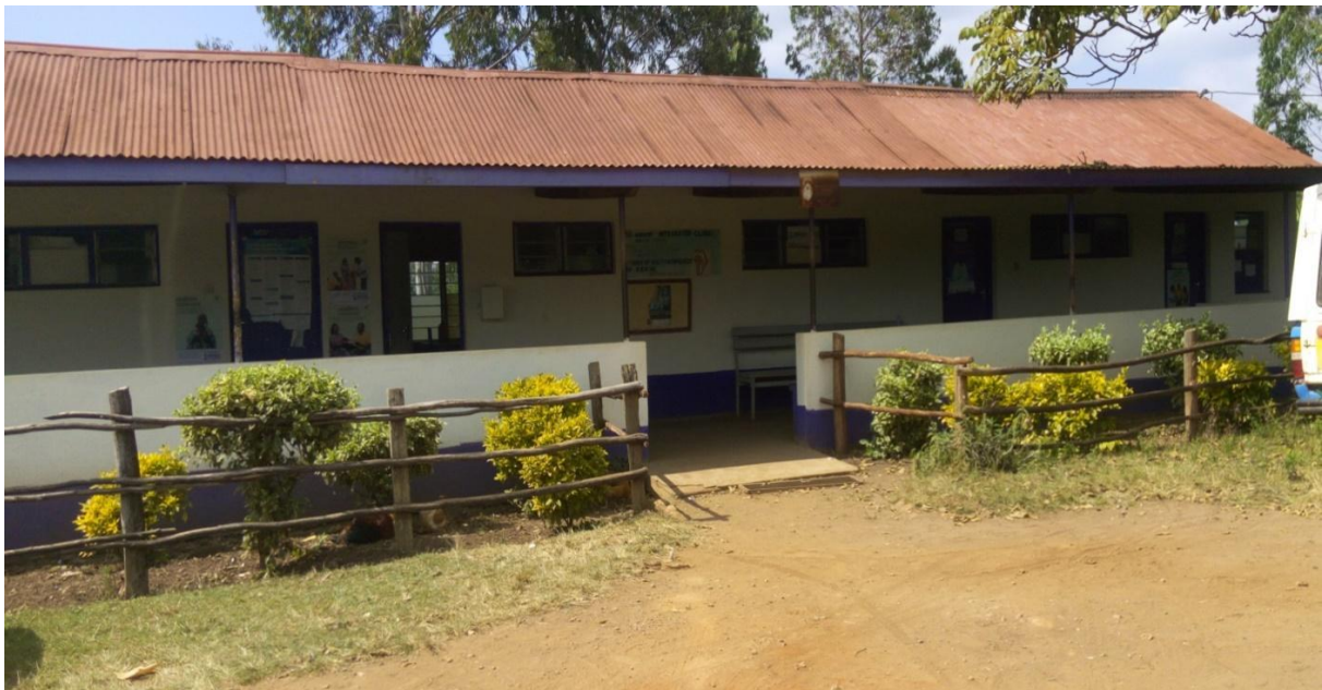
Figure 3.4 A Section of the AIM Dispensary at the Mbooni Mission Station
