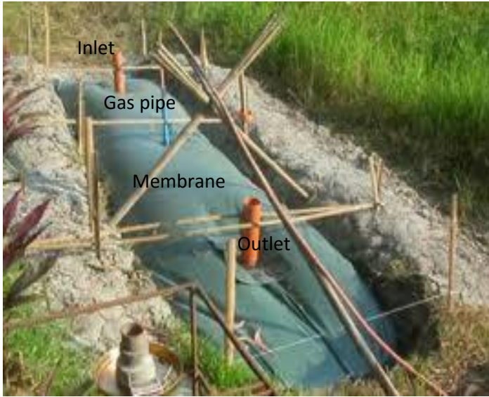
Plate A1.3: Flexible structure
