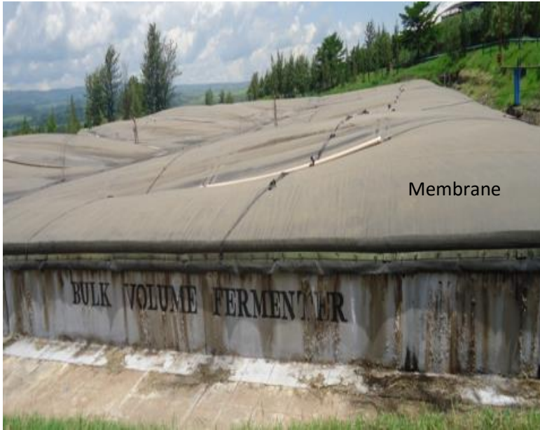
Plate A1.5: Lagoon covered with a membrane
