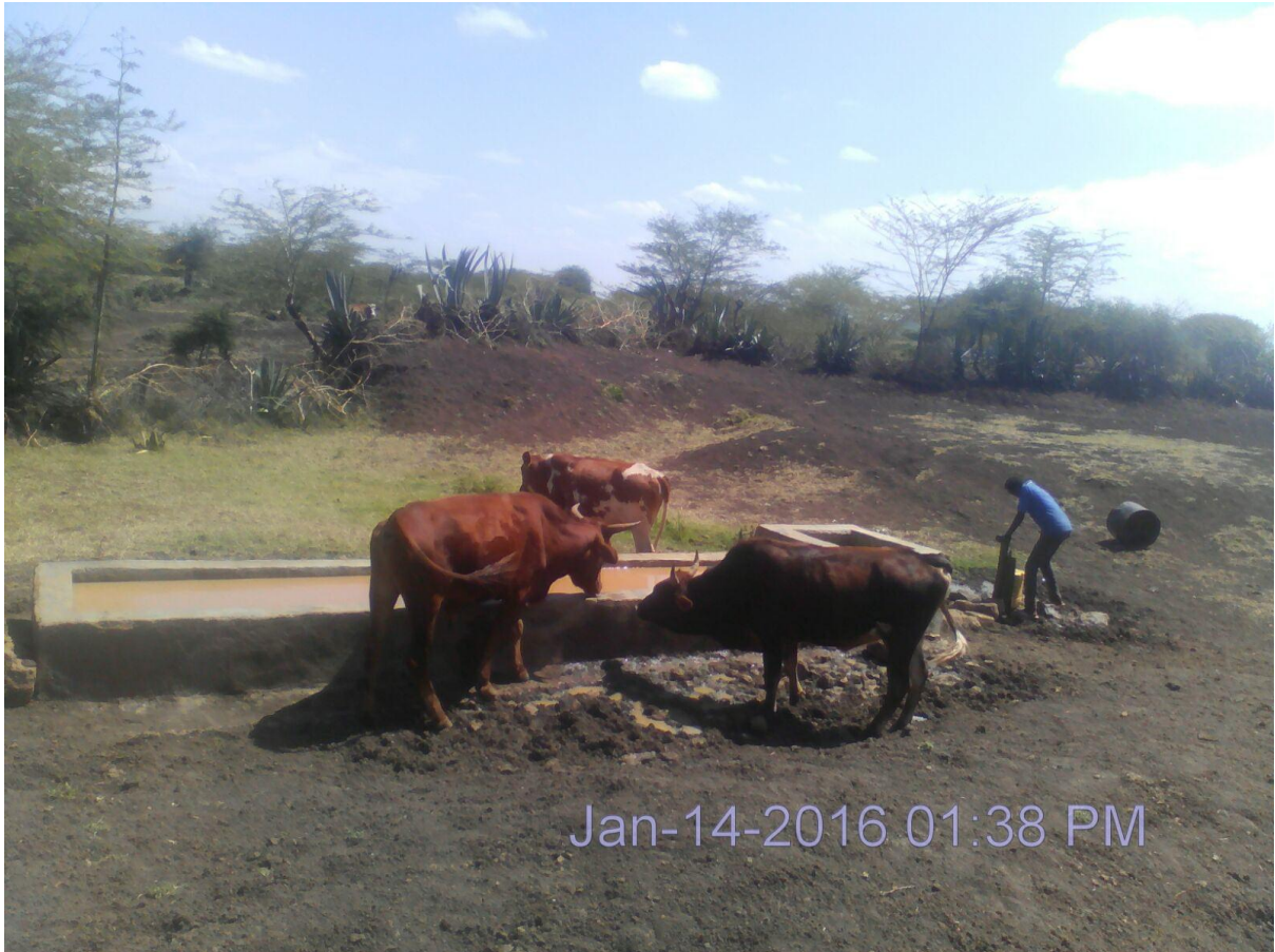
Plate 4.2 : Plates showing Cheraik water pan; Water trough and public standpipe.
