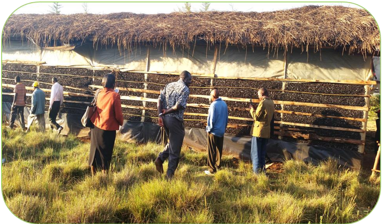
Plate 14: A cold potato storage made of locally available material at Nyaru in Elgeyo-Marakwet County – photo taken by Rael Taiy on 29/9/2015
