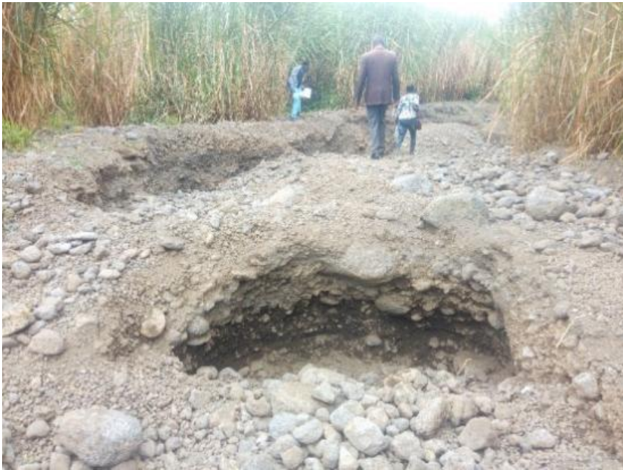
Plate 3. 1. Gully erosion in Gahunga, Burera District
