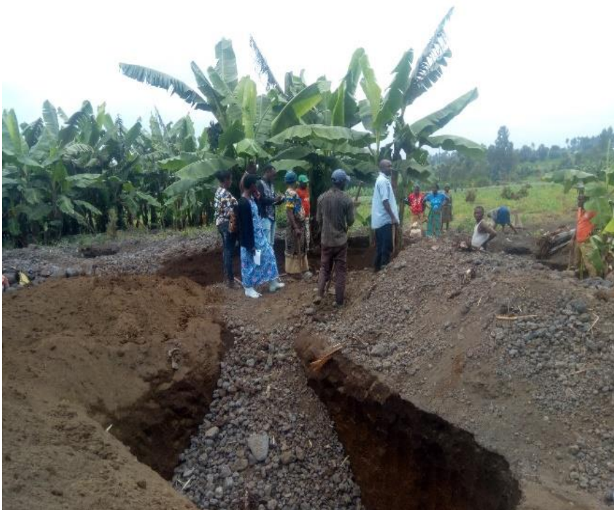
Plate 3. 2. Removing stones that had been transported by erosion from the park
